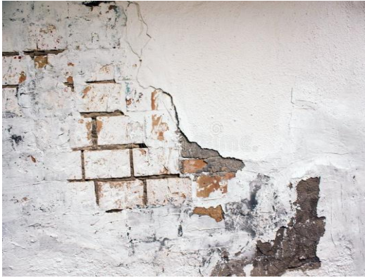
Figure 3.7: Peeling effect on houses
