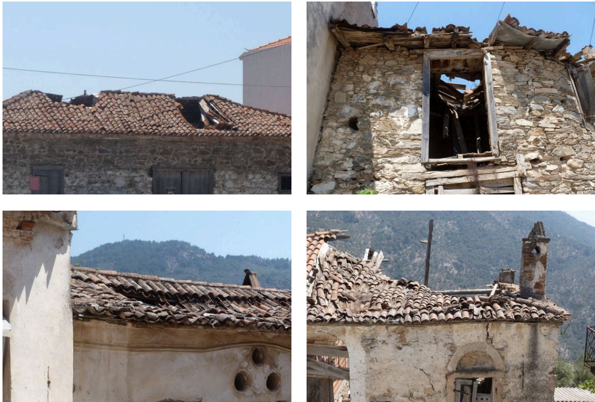
Figure 3.9: Stone houses with collapsing rooftops.
