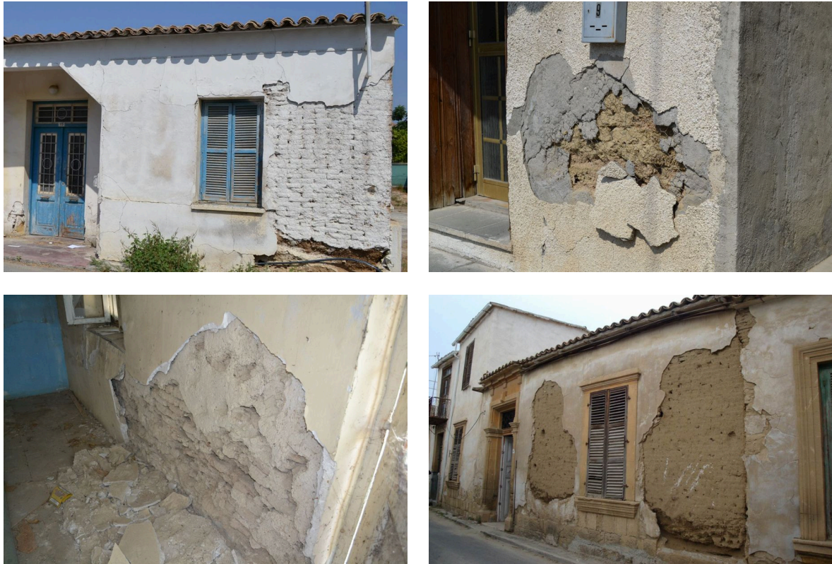
Figure 3.7: Paint and plaster layer is peeled off, revealing the mudbricks.
