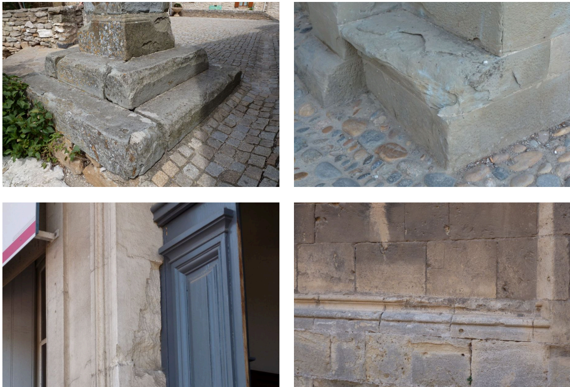
Figure 3.5: Stone structures affected by corrosion.
