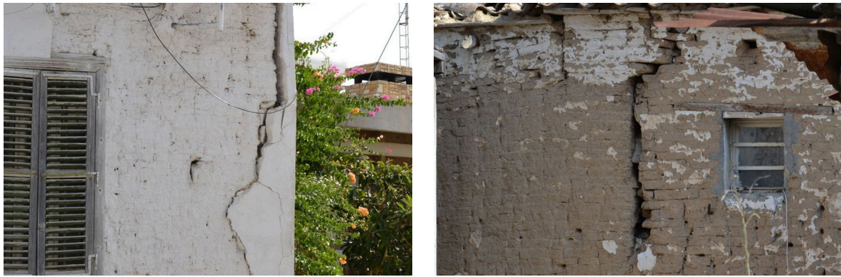
Figure 3.6: Cracks on the walls of mudbrick houses.
