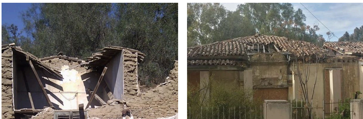
Figure 3.8: Mudbrick house with collapsing rooftops.
