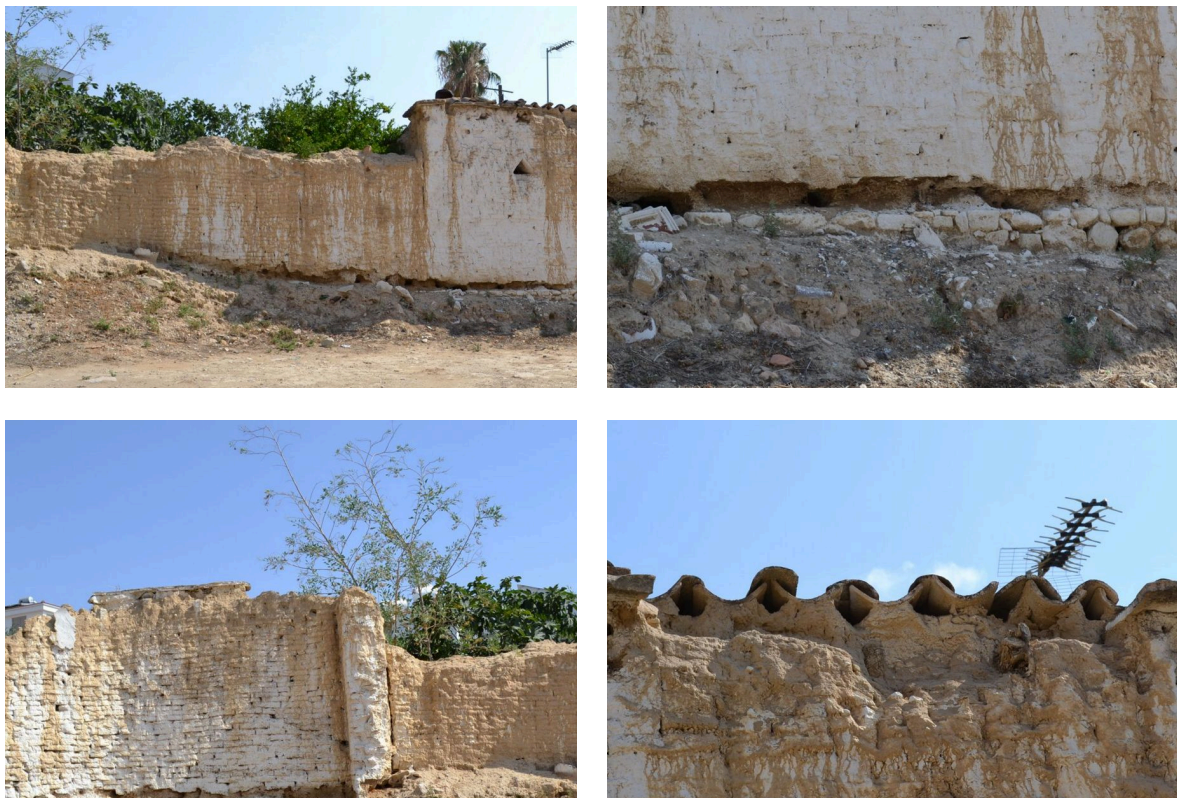
Figure 3.4: Photographs of mudbrick houses subject to corrosion.
